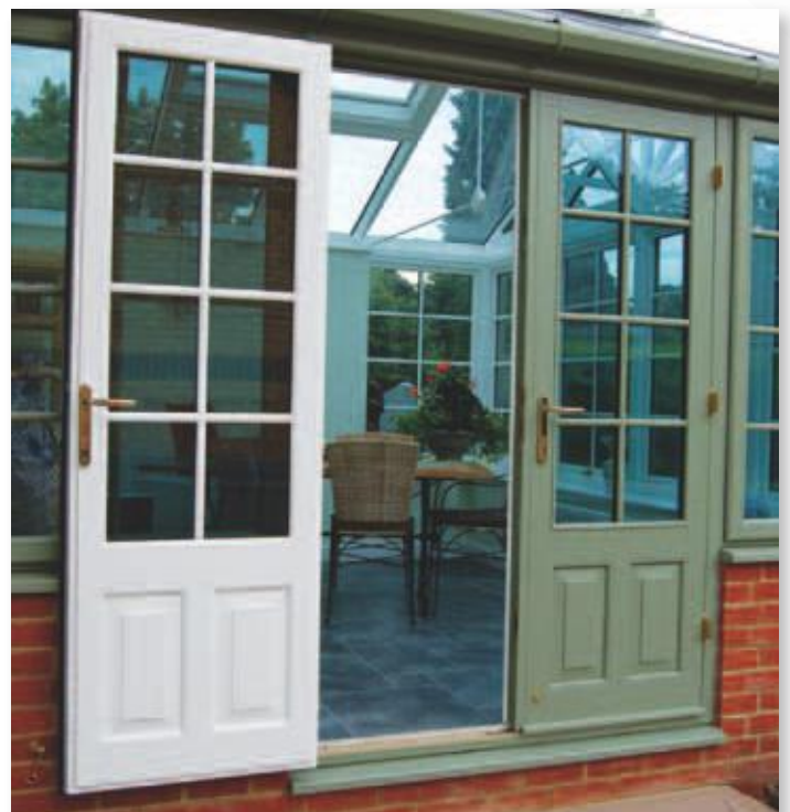
Double doors in a conservatory with locking handles to each door, astragal bars lining through either side and raised and fielded panels below the midrail. The doors are dual colour: green on the outside, white on the inside
