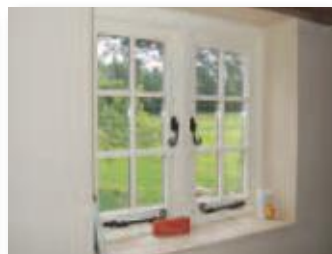
White flush window with astragal bars, monkeytail handles, and a peg stay
